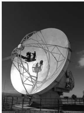
(left) ALMA-NA prototype antenna at VLA site. (right) Working on the panel adjustment for photogrammetry measurement.
