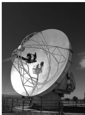
(left) ALMA-NA prototype antenna at VLA site. (right) Working on the panel adjustment for photogrammetry measurement.
